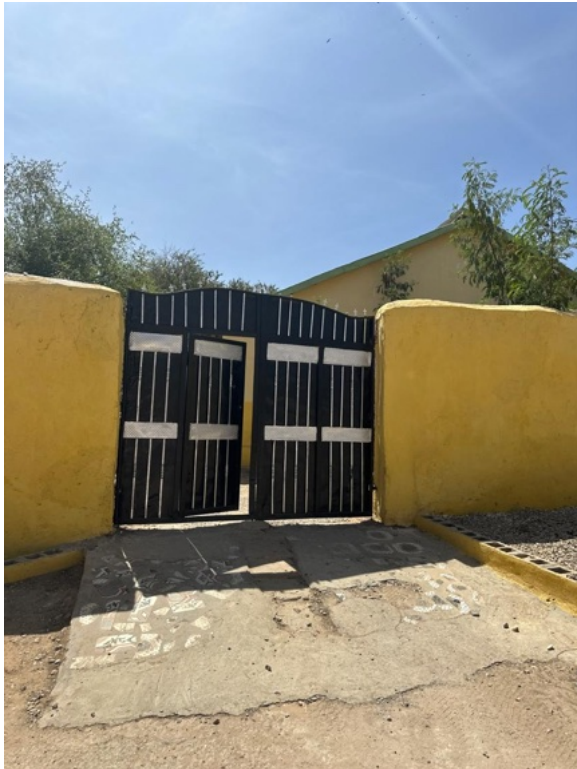
Figure (3.8.2.1): MOFLR main gate
